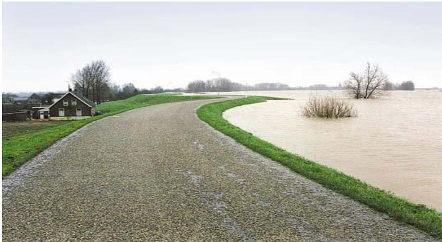
Figure 2.2 Illustration of a river levee in danger of overflowing
